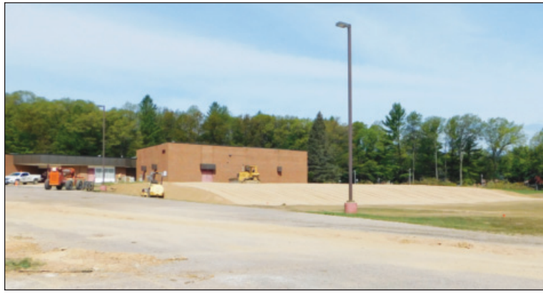
Above left, Larson Elementary as viewed from the southeast last summer. Above right, the structure as it appears now from the same vantage point. Noting the landmark trees in the background lends a sense of the project's scale.
